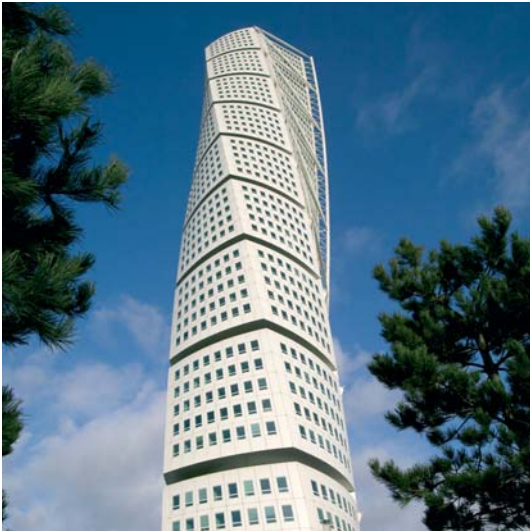
Turning Torso, Malmö, Sweden
